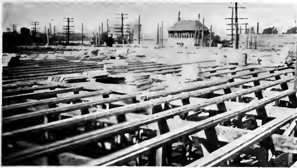
FLOOR FORMS UNDER CONSTRUCTION
